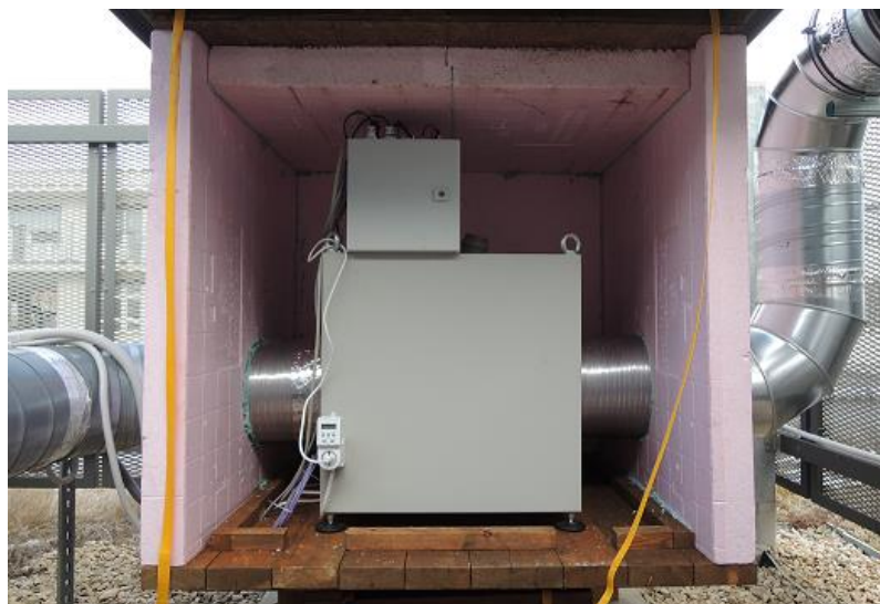
Installation of PET-02 in air ducts in a nuclear medicine facility
